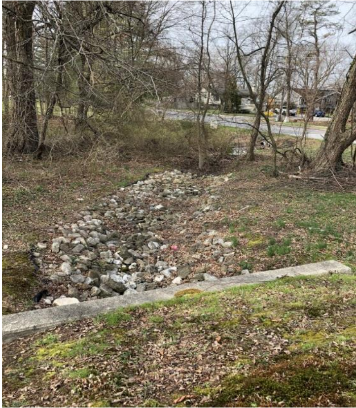
SWM pond outfall into Reach 1 from embankment
