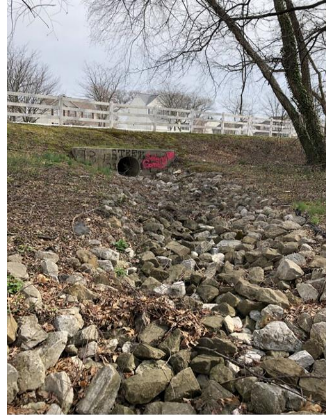
View of SWM pond outfall from below
