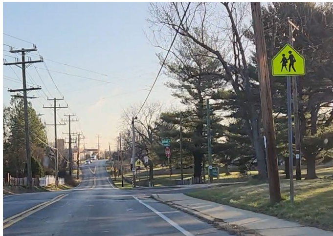
Figure 4: Duplicate advance school crossing signing for Washington Avenue crosswalk
