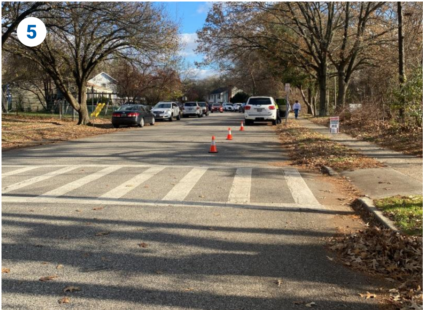
Crossing Myers Drive at Stafford Hill Drive
