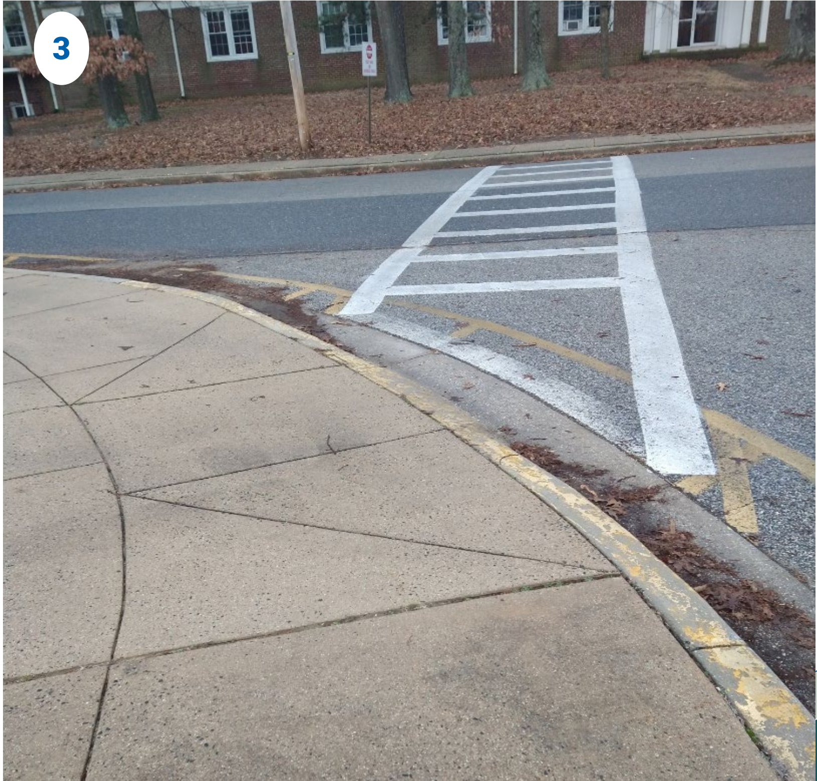
Crossing the entrance to the bus lane and parking lot.
