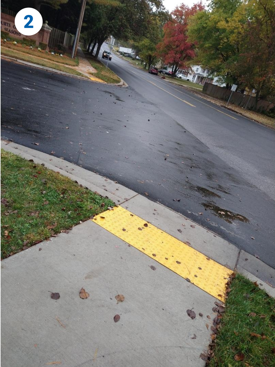
Crossing of Summer Hill Drive.
