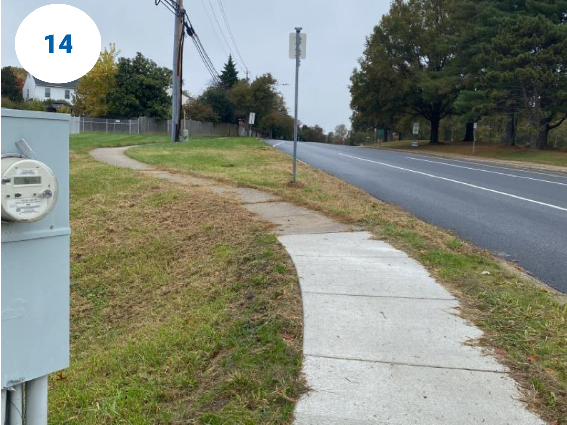
Steep cross slope along the sidewalk on Waugh Chapel Road.
