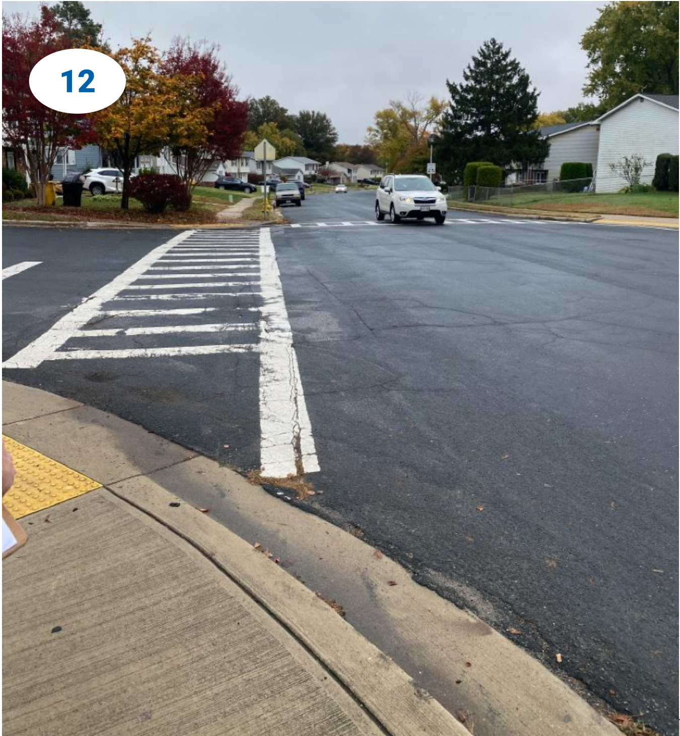
Intersection of Maytime Drive and Springhill Way.
