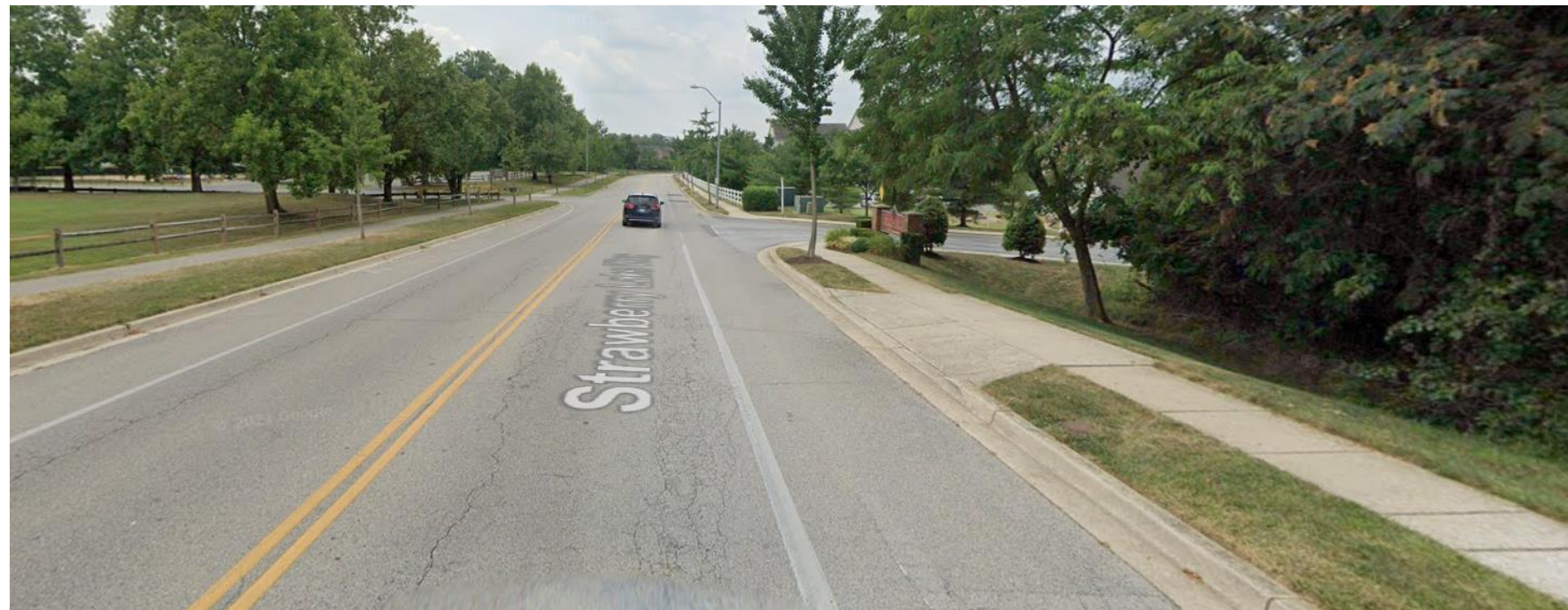
View of Strawberry Lake Way near GORC Park via Google Maps
