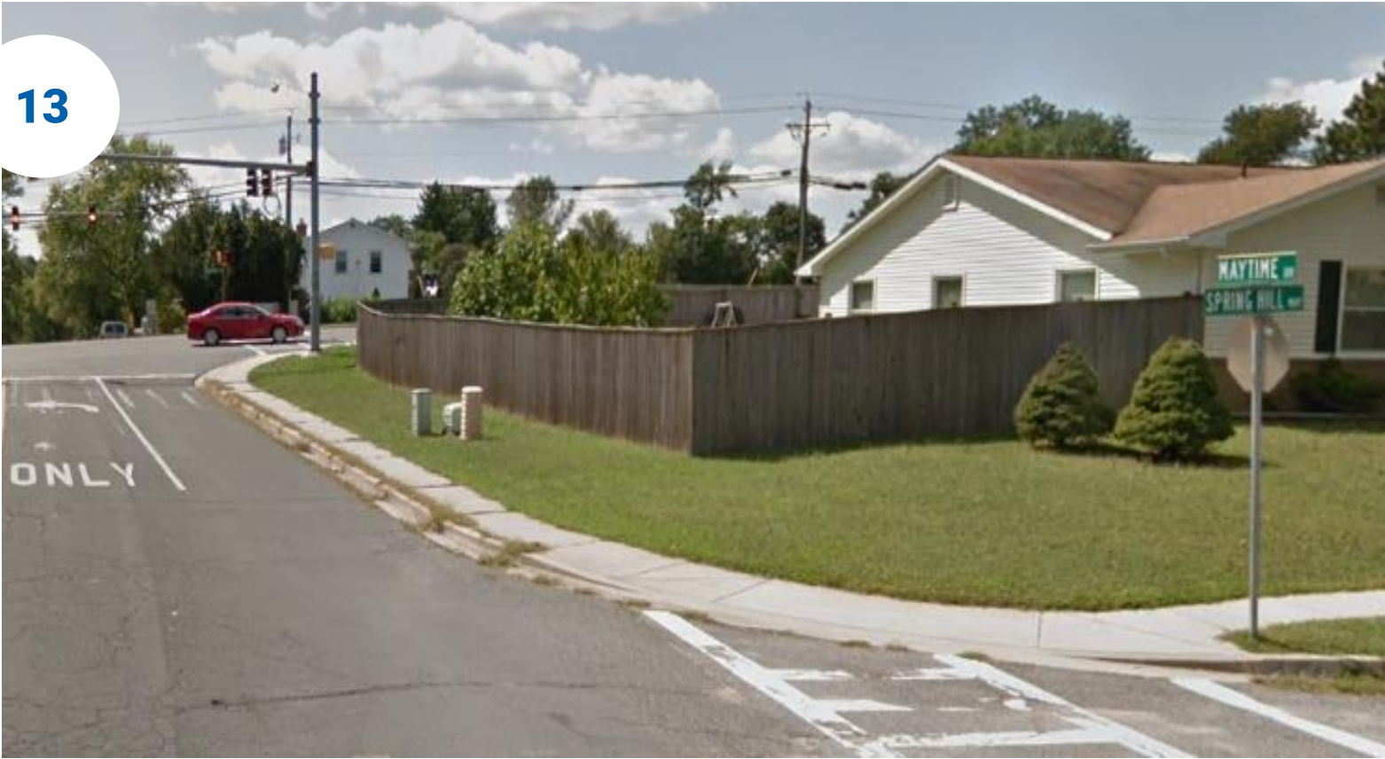
Sidewalk on the north side of Maytime Drive.
