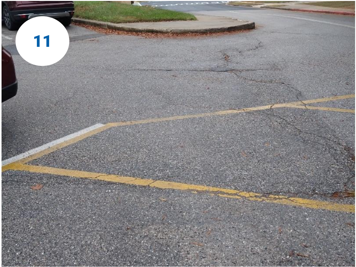
School parking lot with view of eastern sidewalk.
