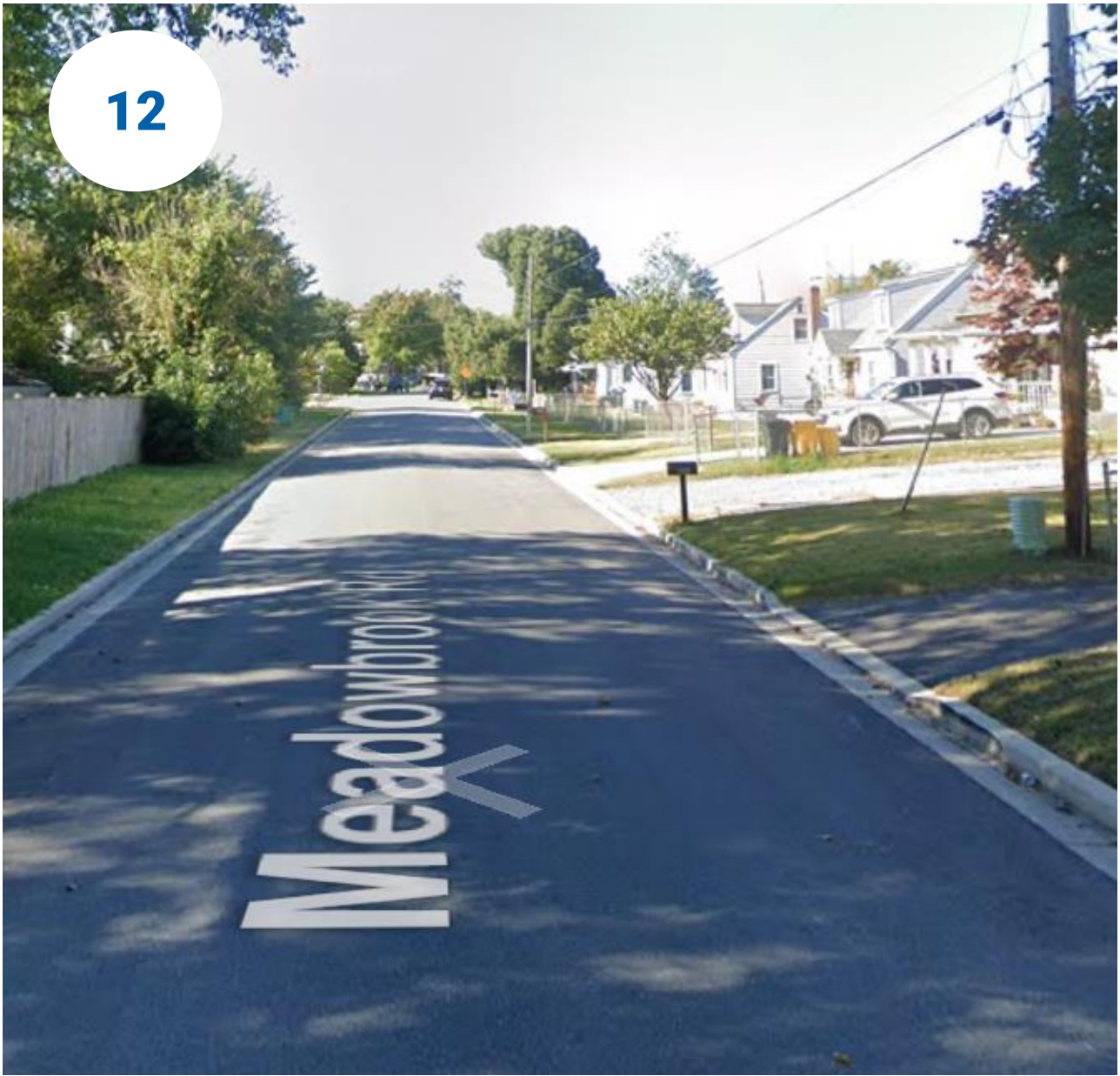
Meadowbrook Road, looking west
