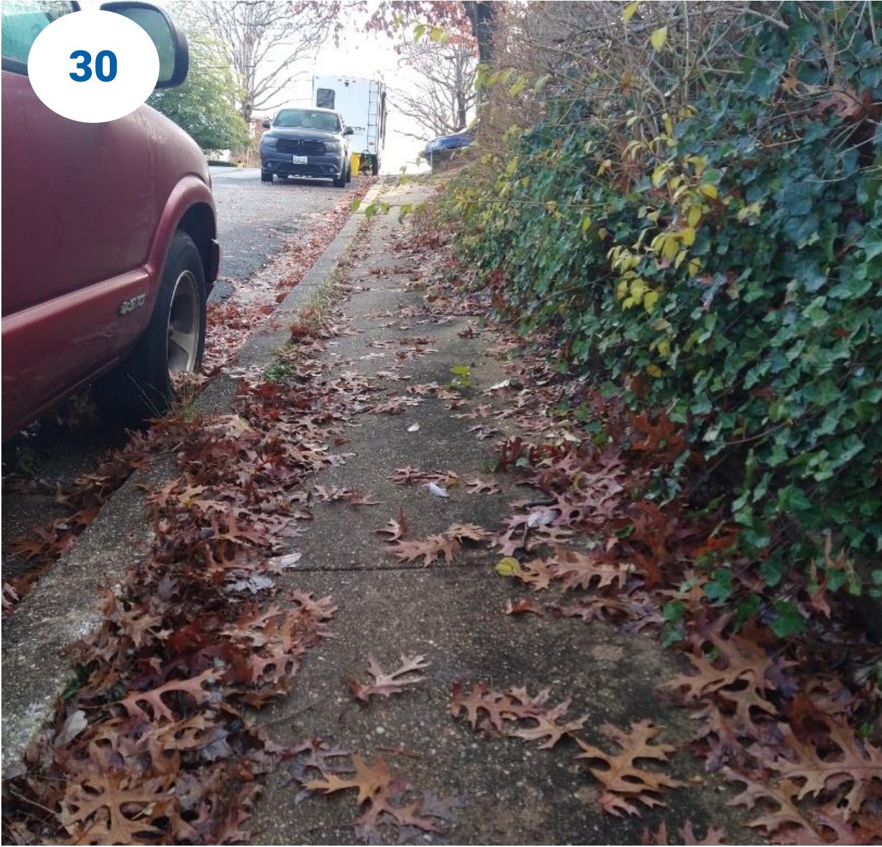
Existing sidewalk segment on 17 th Avenue
