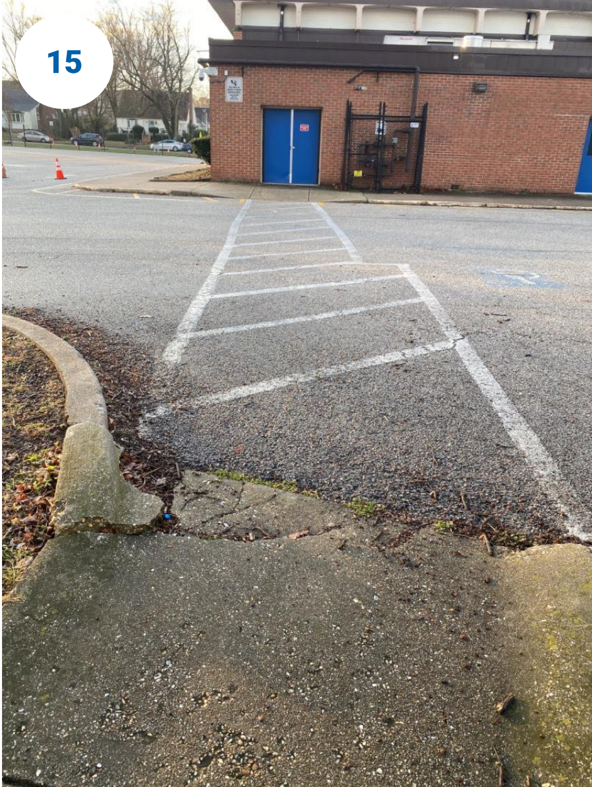
The crossing over the parking lot to the walker entrance
