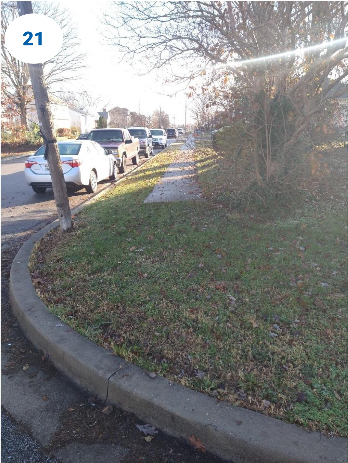
15h Avenue where the existing sidewalk begins
