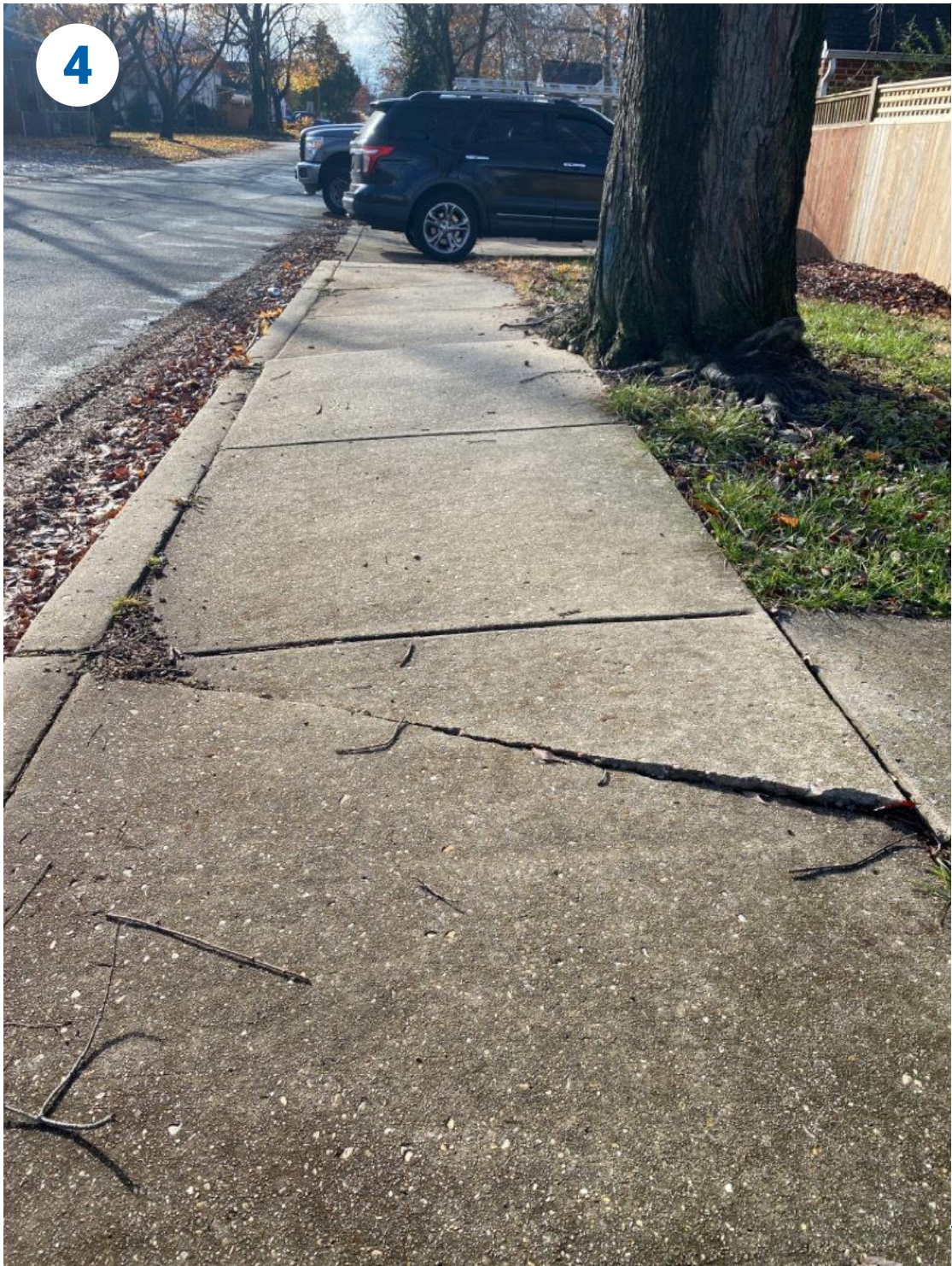
West sidewalk on Marshall, just south of 10 th Avenue
