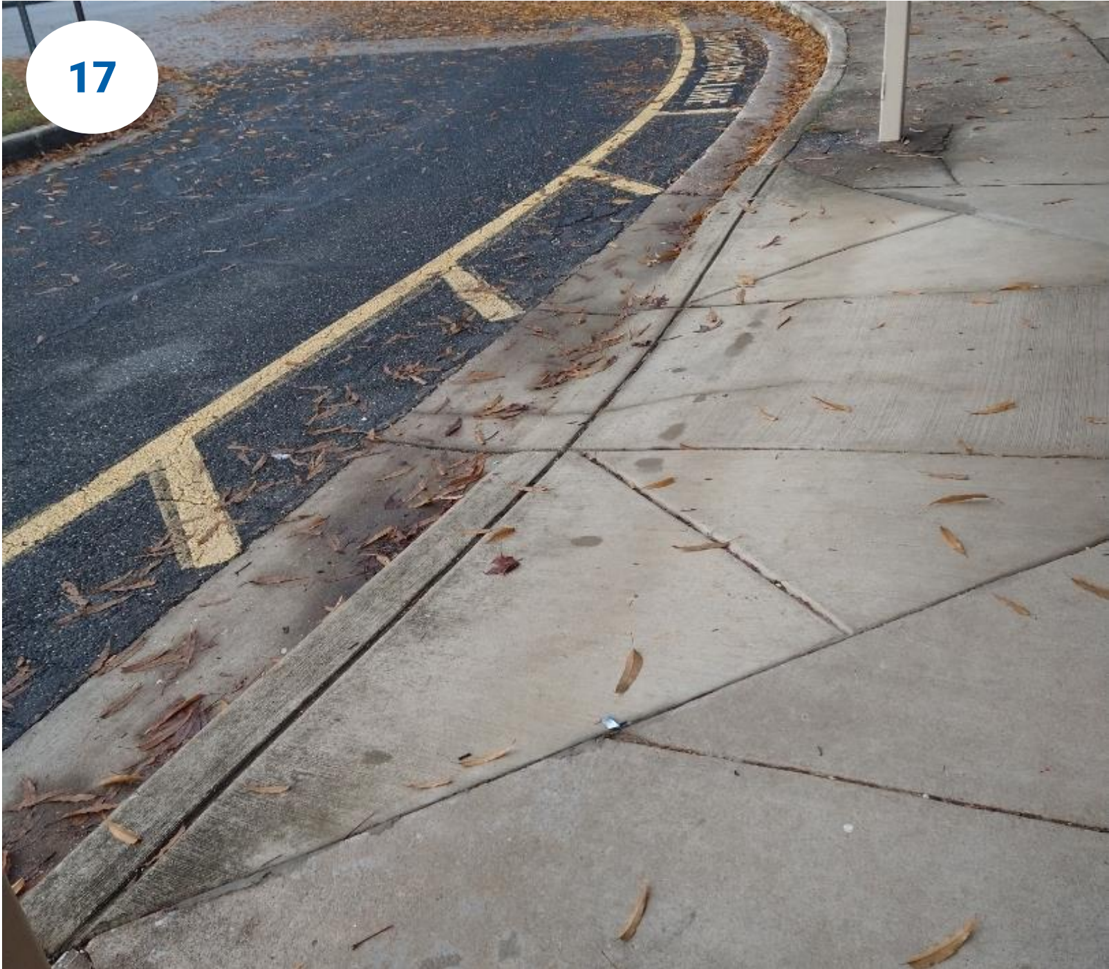
The curb ramp at bus drop off
