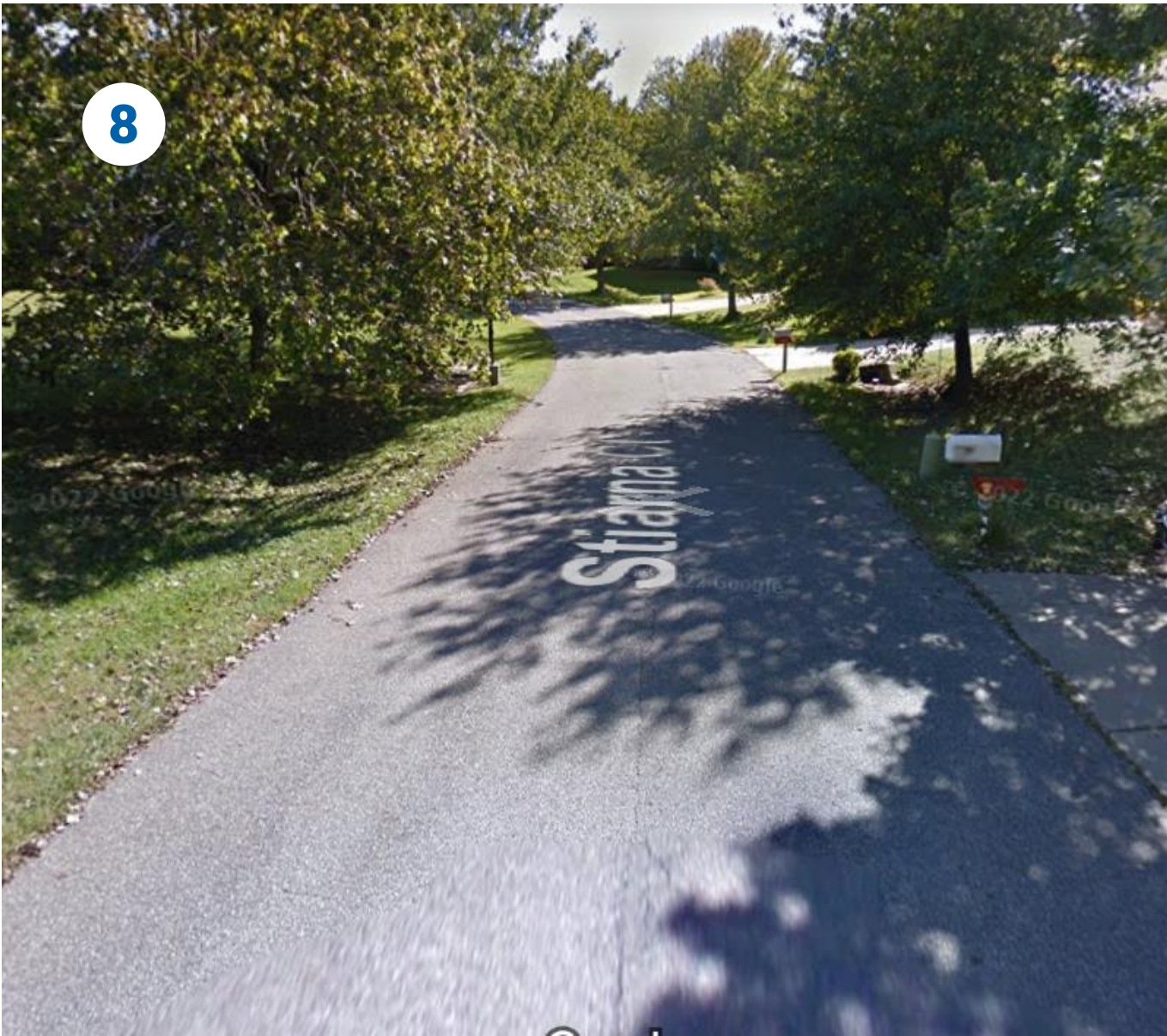
Stiarna Court – missing sidewalk
