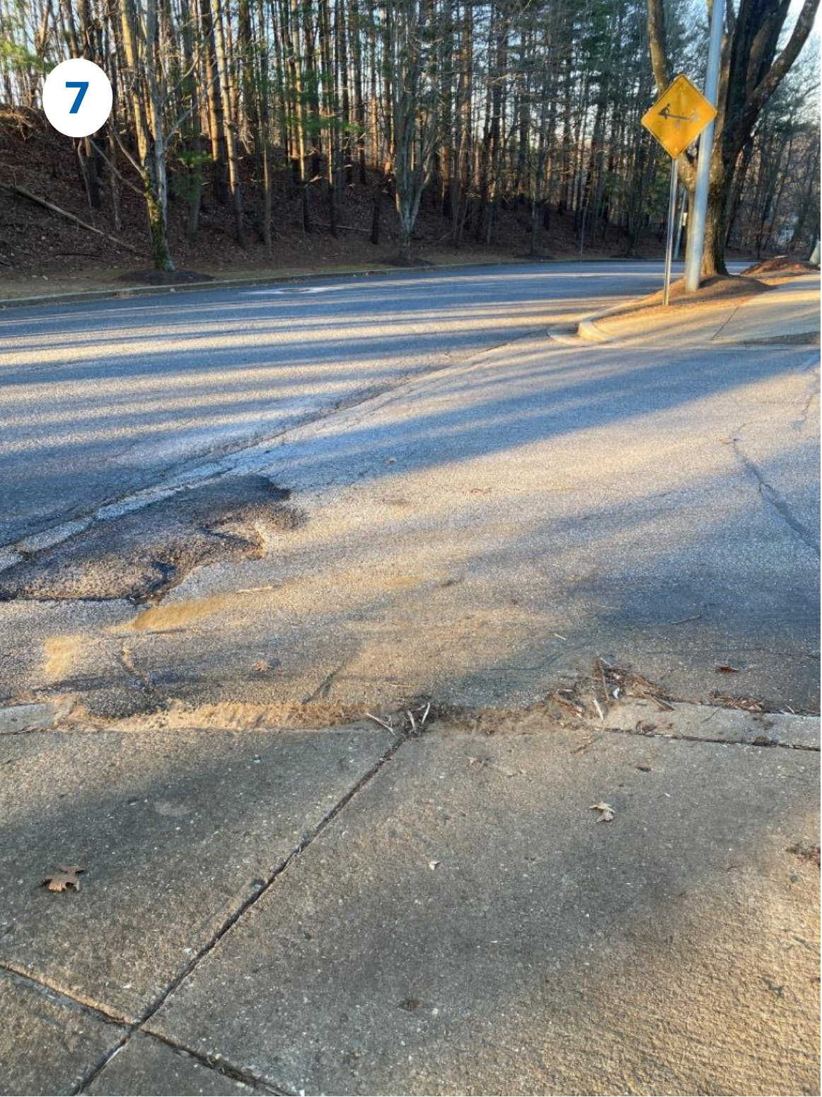
Crossing Palmwood Court at Greenhill Road
