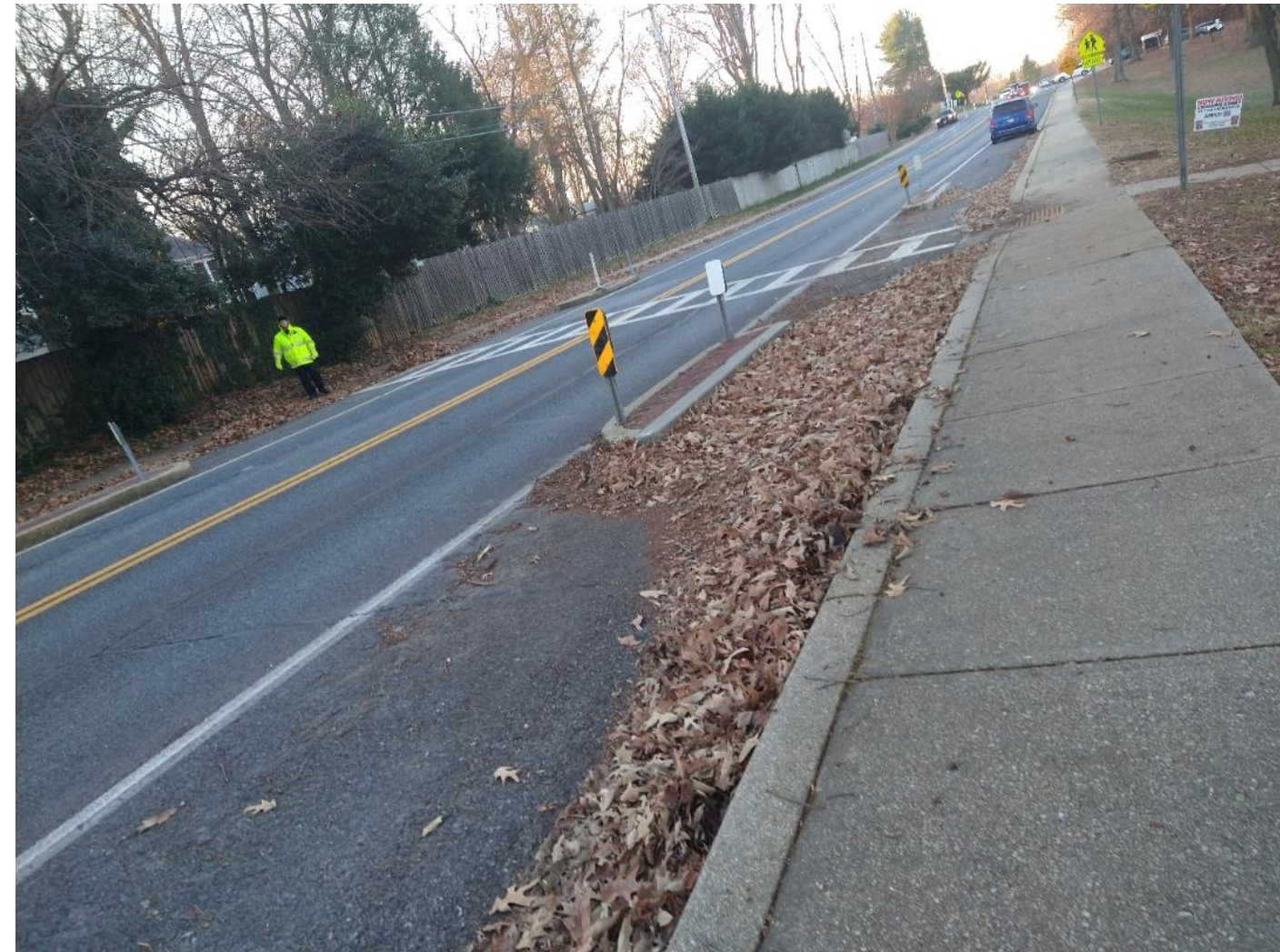
Shore Acres Road - midblock crossing guard
