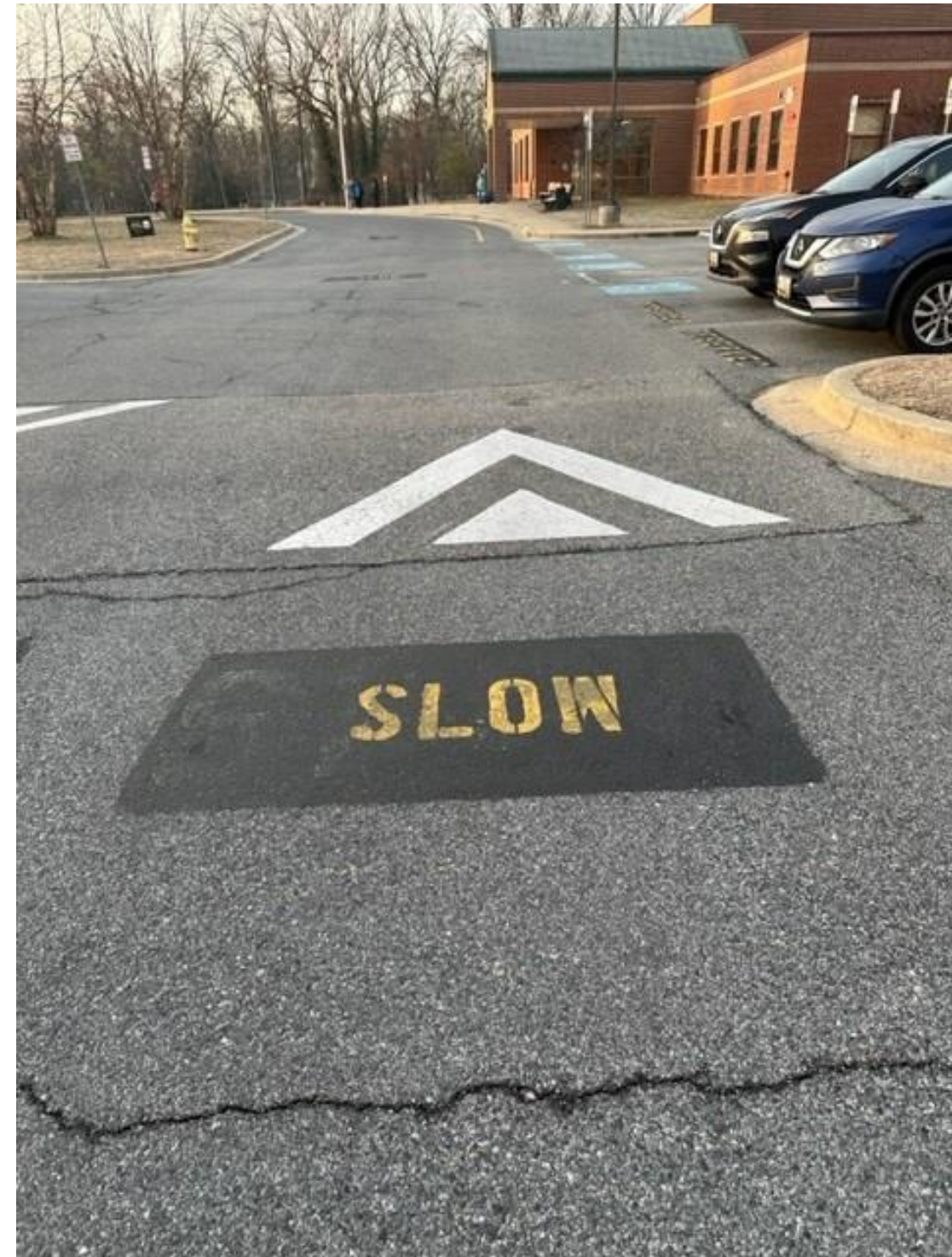
Several speed humps are installed in the parking lot/drop-off loop.
