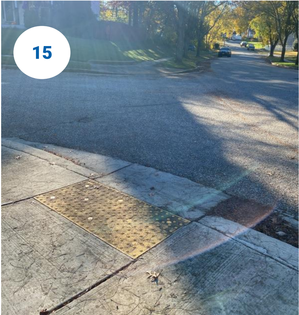
The crossing of Snow Valley Lane and Snowfall Court
