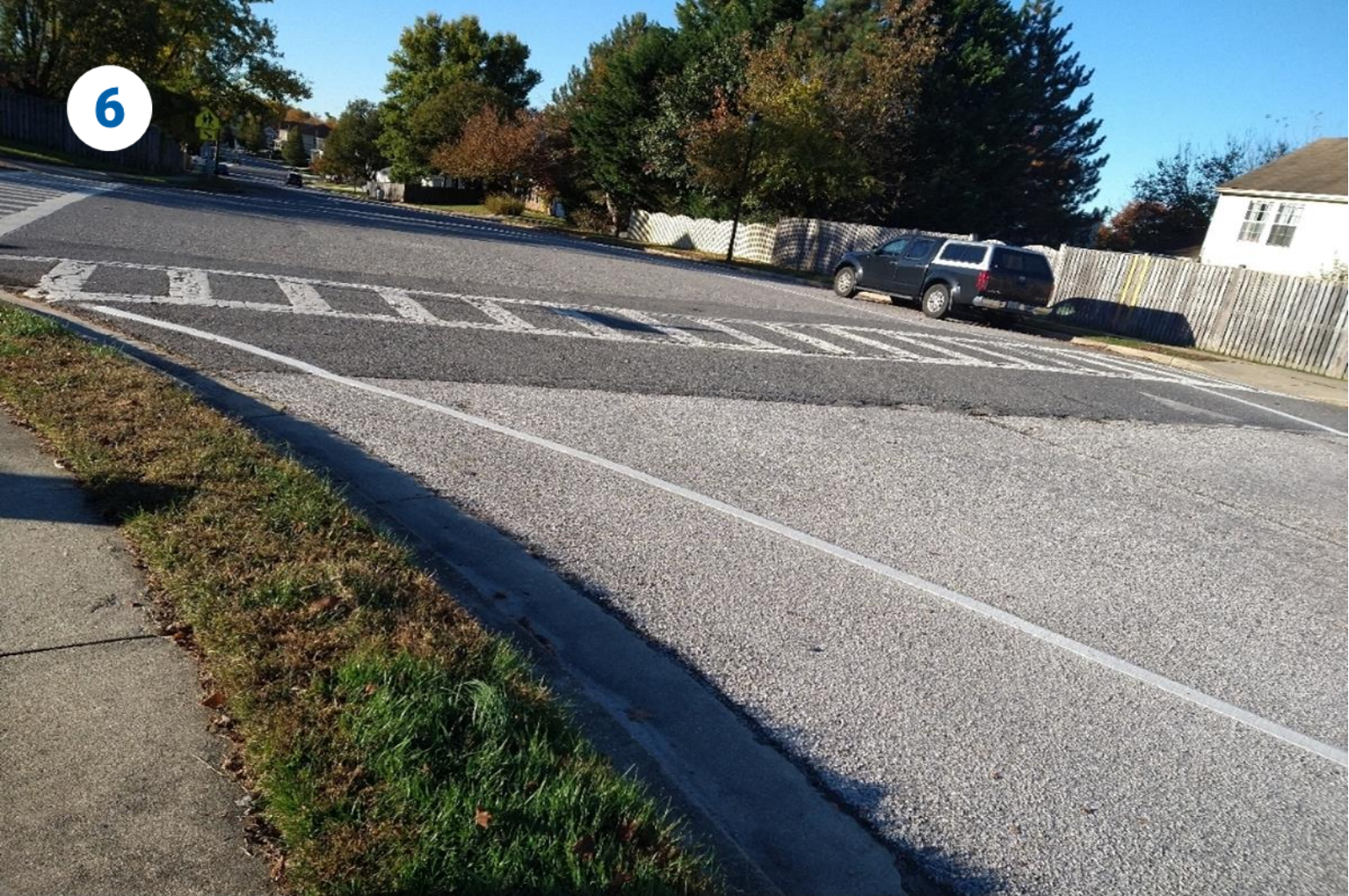
The raised crosswalk at the intersection of Indian Summer Drive and Sunflower Drive.
