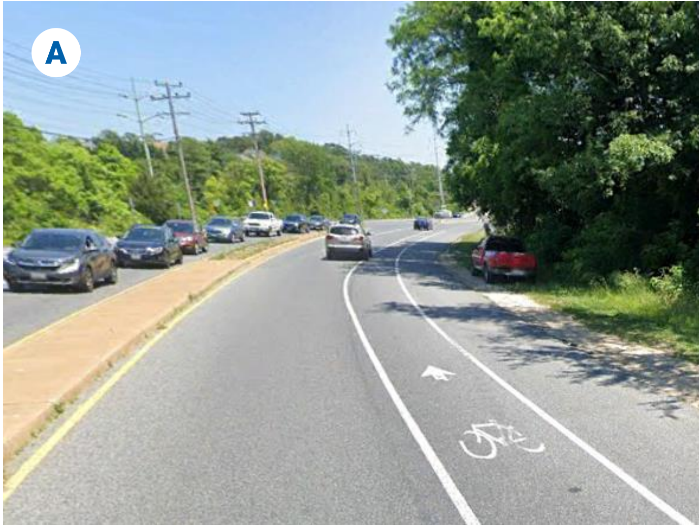
North Camp Meade Road looking north of Valley Road
