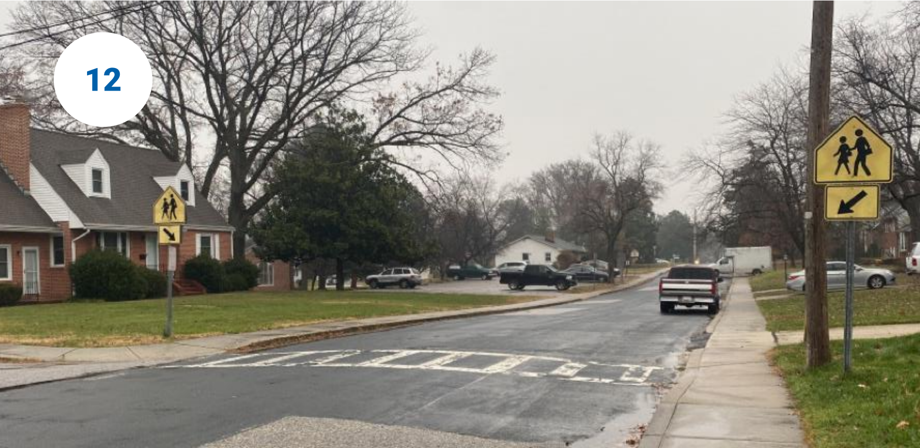
Crossing School Lane at Linthicum Heights United Methodist Church driveway
