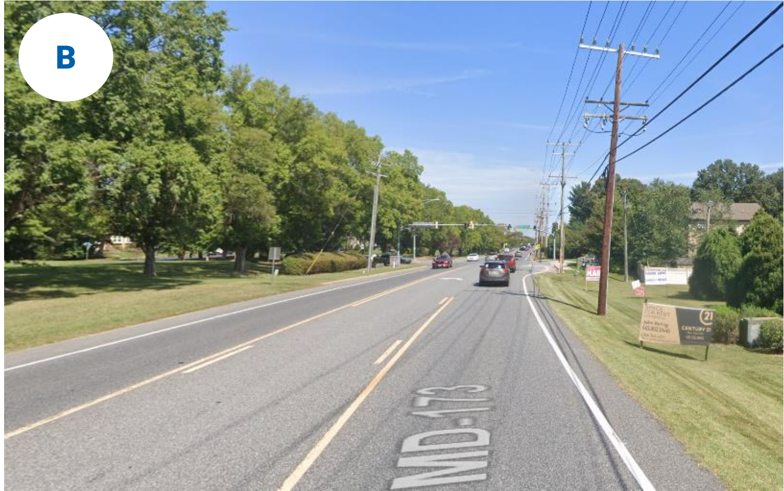
Fort Smallwood Road (MD-173), approaching the school campus
