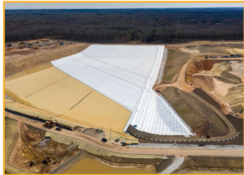
Landfilling in Subcell 9.1, construction of Subcell 9.2, 2021
