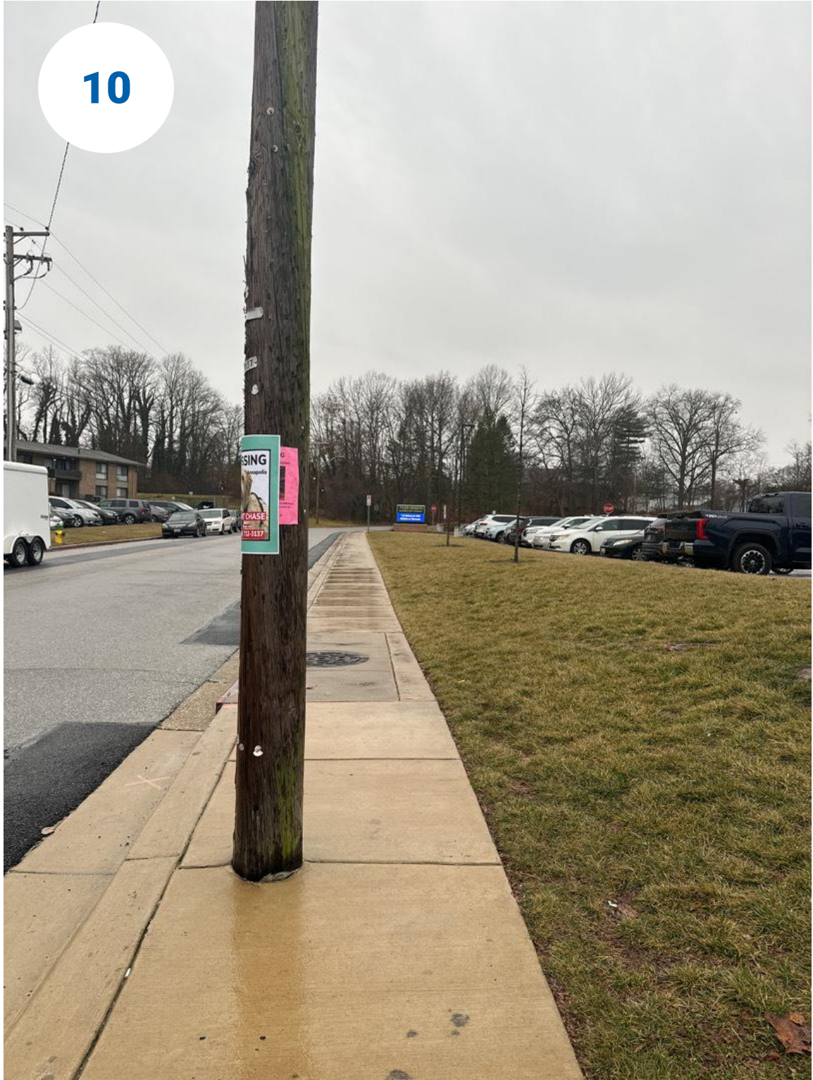
Sidewalk obstruction on Janwall Street
