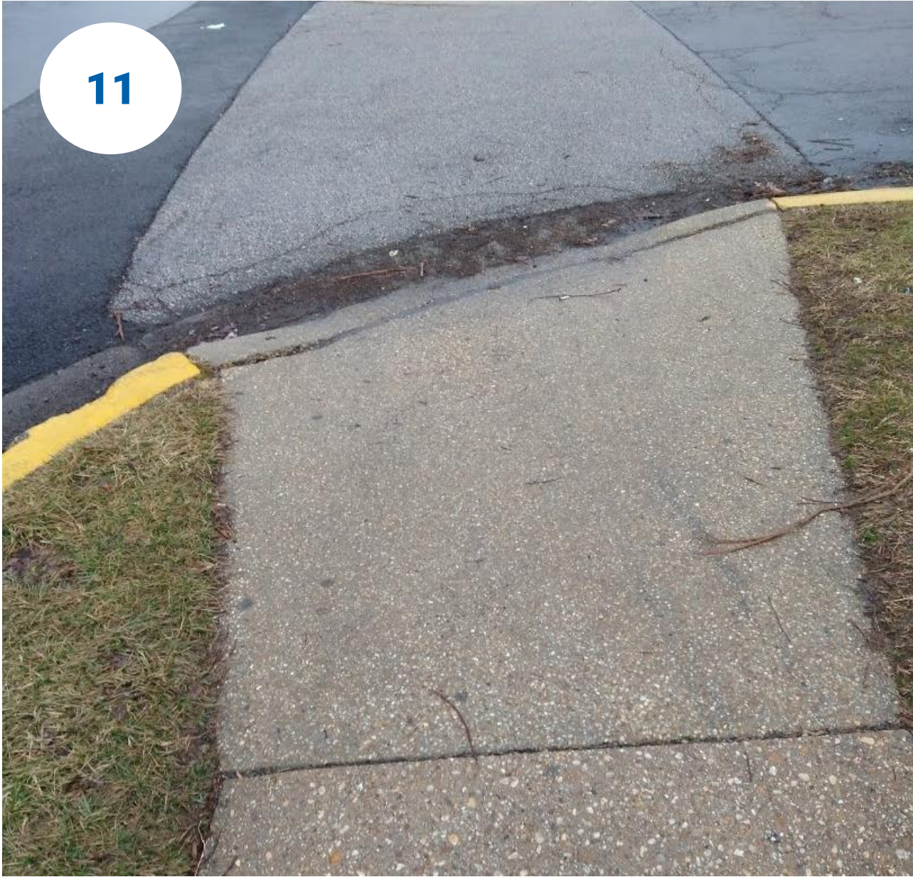
Bricin Street & Apartment Parking
