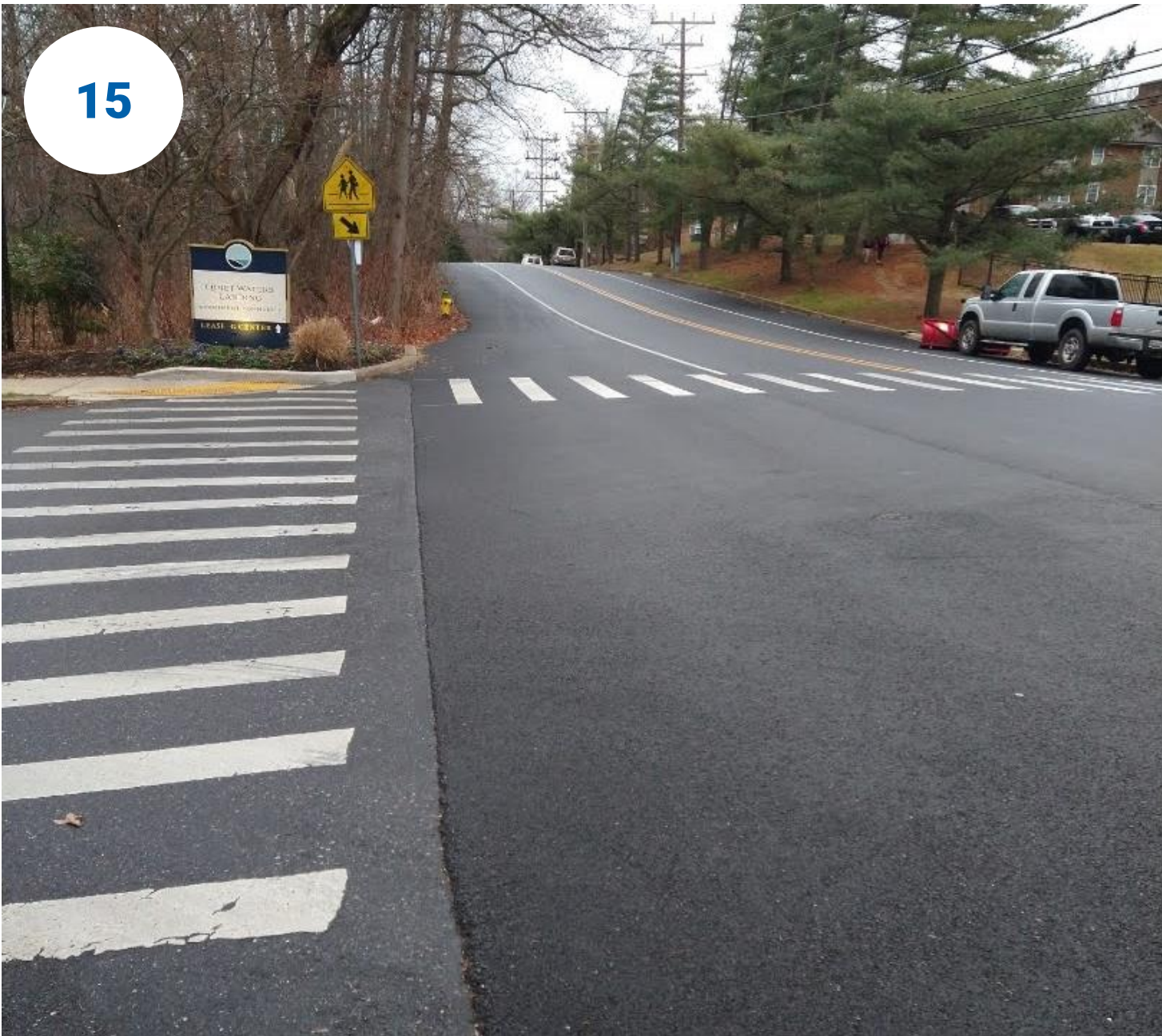
Bricin Street & Forest Hills Avenue
