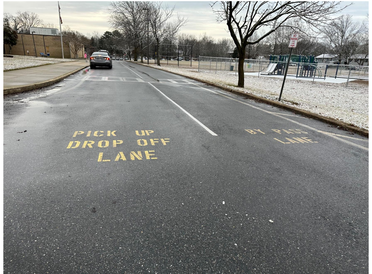
Pavement markings on the school driveway for parent drop off and pick up.
