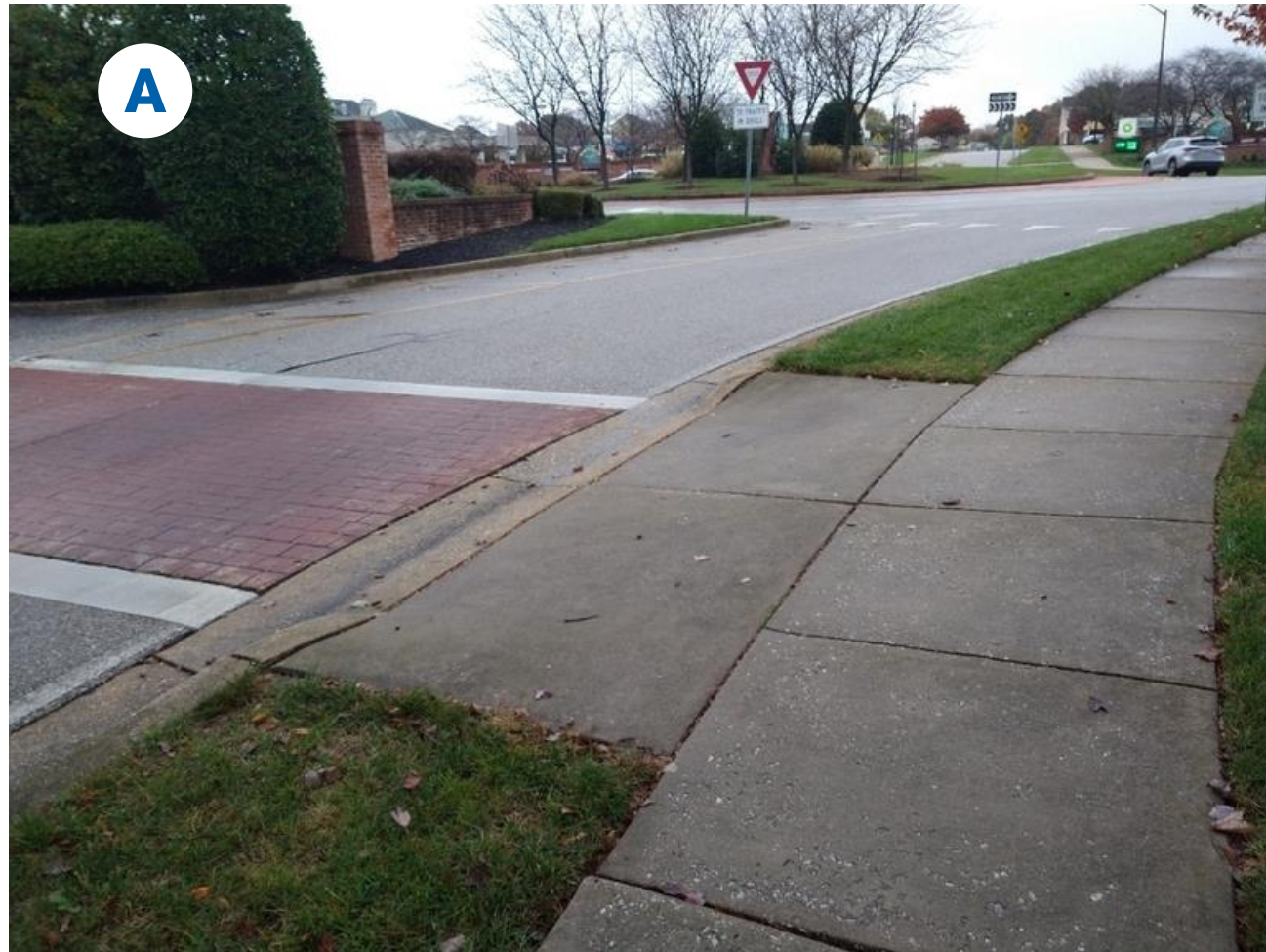
Crossing Roaming Ridge Way; the roundabout at Piney Orchard Parkway is in the background.
