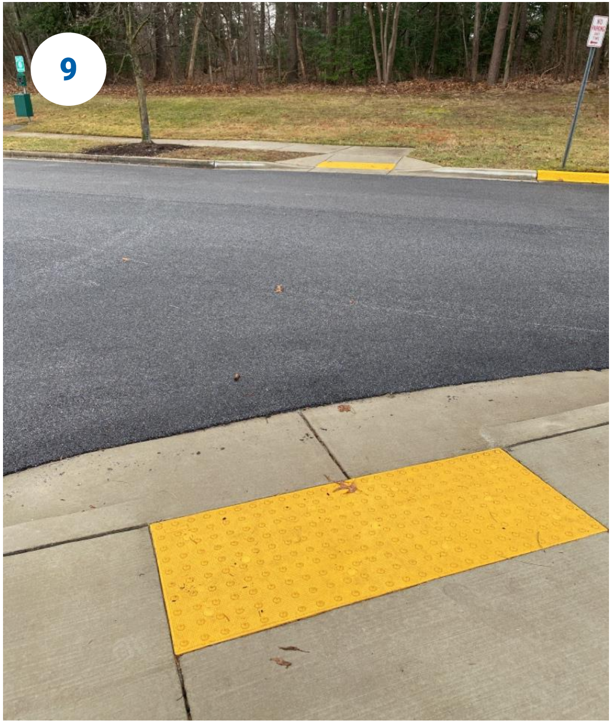
Crossing Willowby Run at end of east sidewalk
