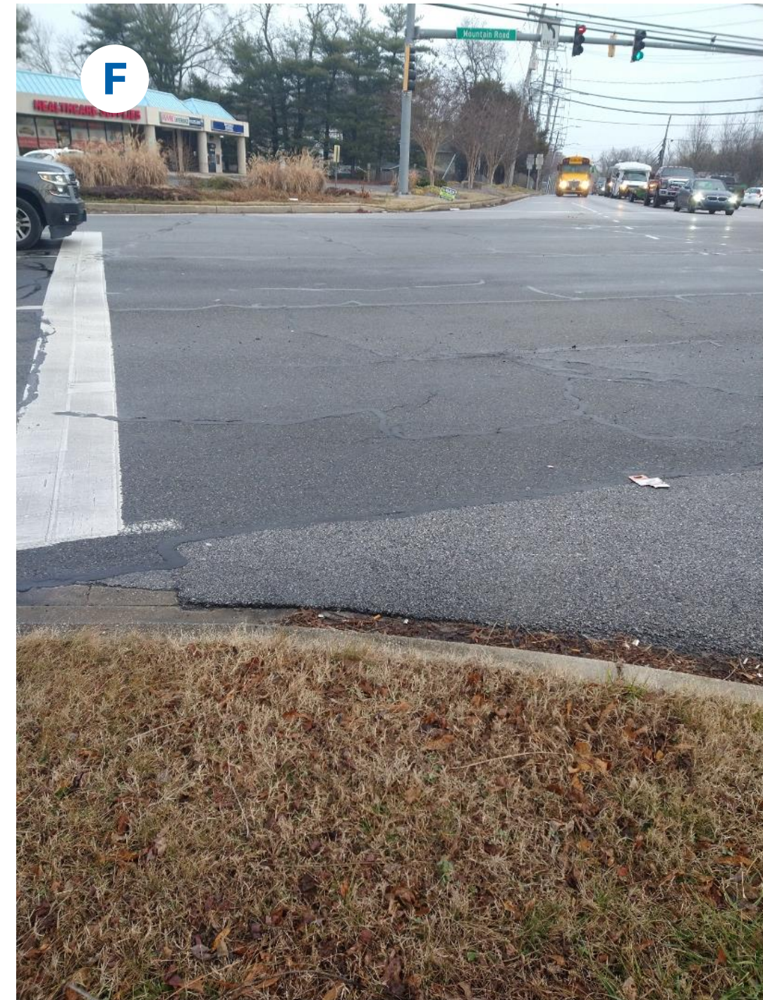
Mountain Road crossing at Hog Neck Road/ Magothy Bridge Road
