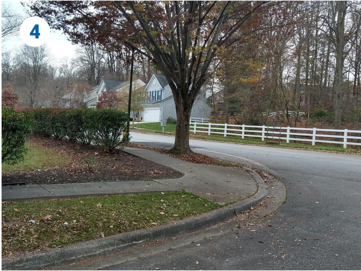
Many of the side streets intersecting with Chelmsford Drive lack marked crosswalks and detectable warning surfaces on the curb ramps.
