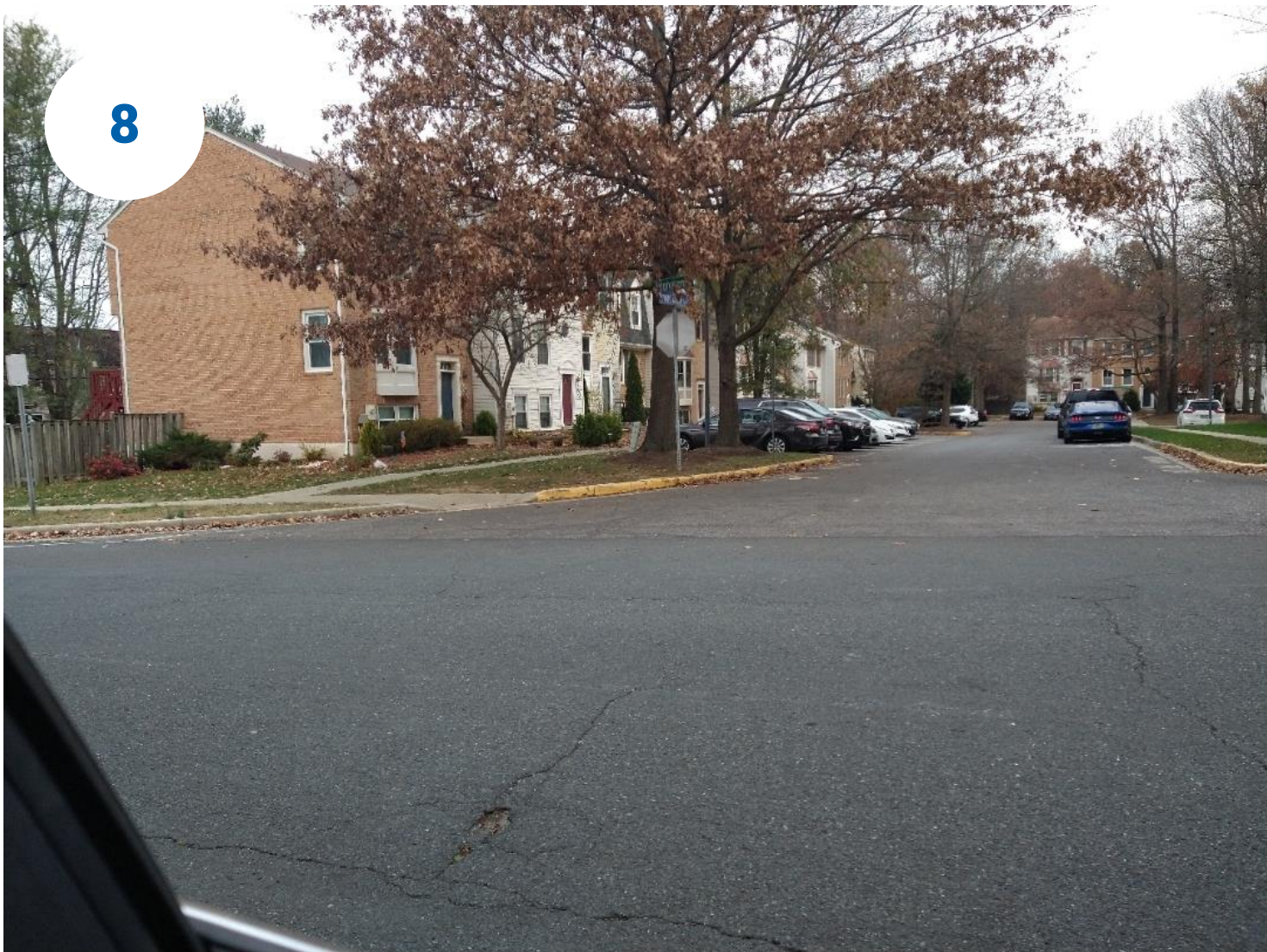
Tilghman Drive at Howard Chapel Court – part of recommendation corridor.
