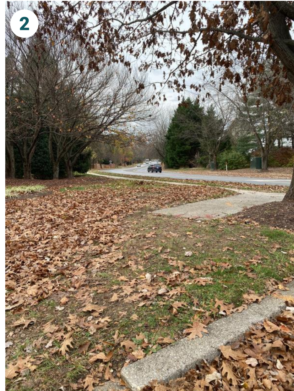
A gap in the sidewalk on Chelmsford Drive near Riedel Road.
